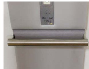
Straight stainless steel handrail
